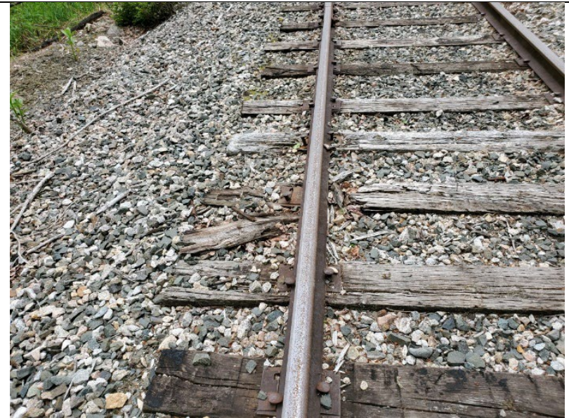
Concord-Lincoln Corridor, Lincoln/Woodstock area Timber Railroad Ties Installed 1931
