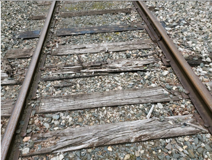
Groveton Branch, Jefferson/Lancaster area Timber Railroad Ties
