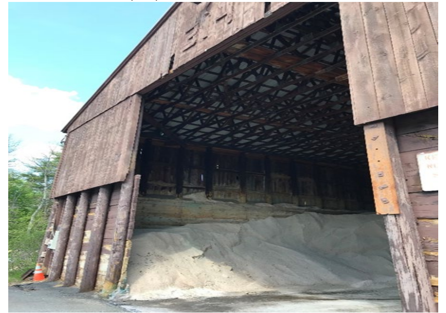
Photo 4 – Belmont (314) – Salt Shed Entrance
