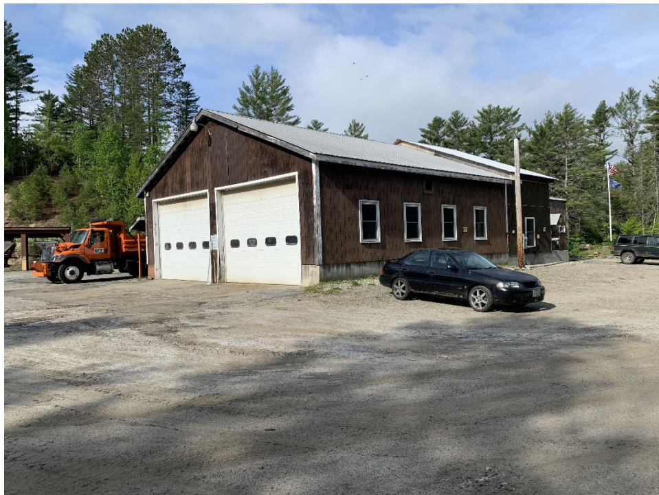
Truck bay exterior
