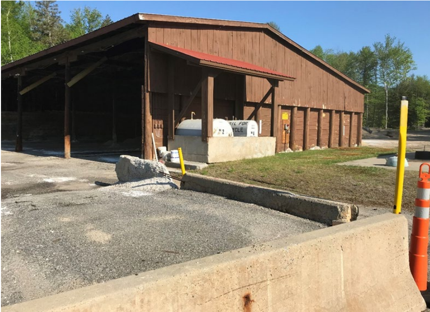
Photo 1: Lincoln (115) – Salt Shed and Loading Ramp
